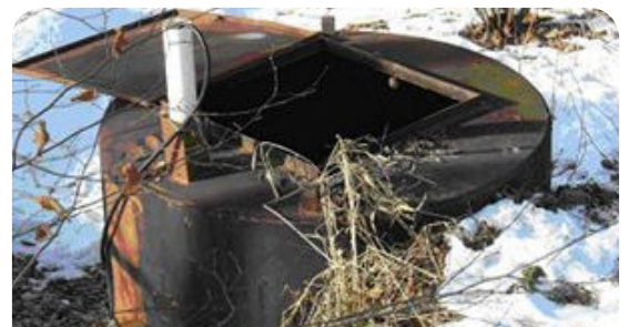
Fig. 2: Vertical steel tank disposal vessel
