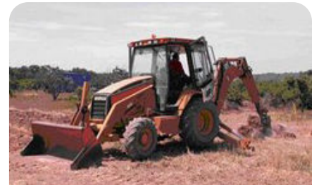
Fig. 7: Backhoe for digging burial trench
