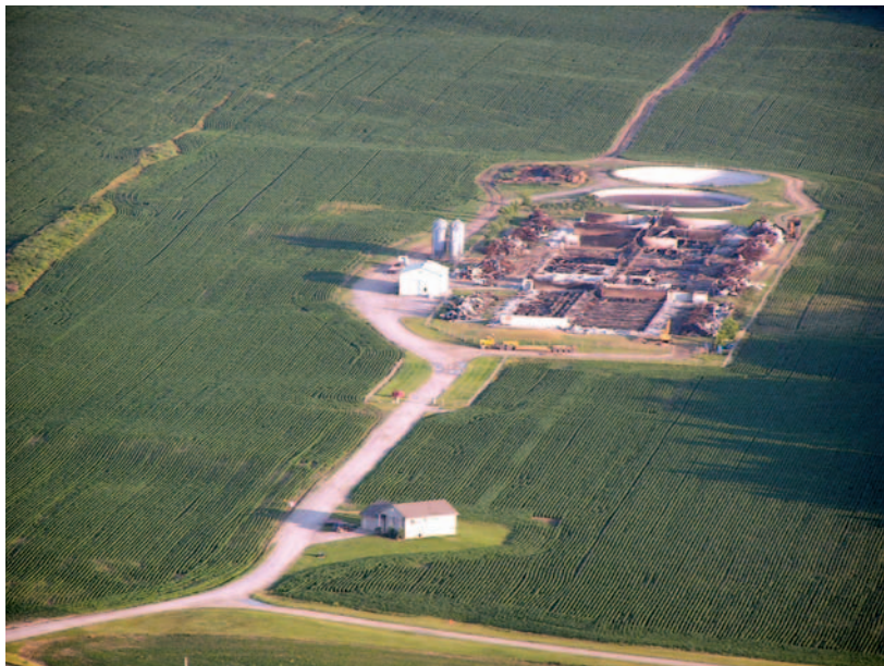
Figure 4.2. This swine facility was devastated by a fire. Note the lack of an access road completely around the buildings which hampered the ability to fight the fire.
