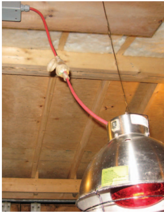
Figure 3.13. The heat lamp is connected directly to a wet-rated electrical box and includes a wet-rated cord cap connection so the lamp fixture can be removed. When the lamp is removed, the cover is placed on the female cap end to protect it from corrosion.
