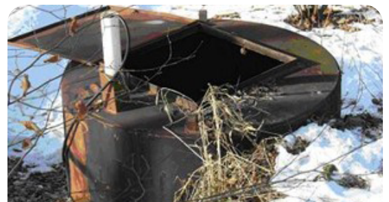
Fig. 2: Vertical steel tank disposal vessel
