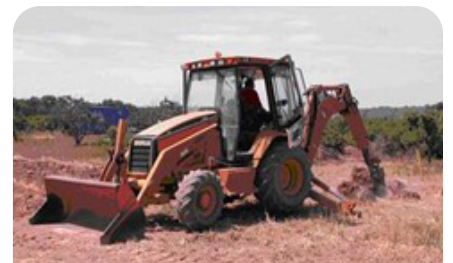
Fig. 7: Backhoe for digging burial trench
